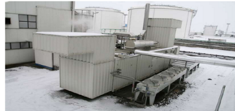
Fig. 51. View of a cogeneration system with an electrical output of 1.5MW and a thermal output of 1.7MW
