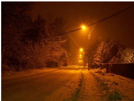
Fig. 44. A road illuminated by means of luminaires with a sodium source
